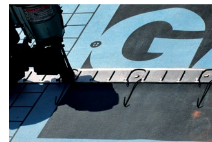
Install Battens & Hangers
