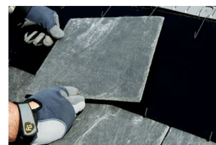
Insert UV & Moisture Barrier And Field Slates
