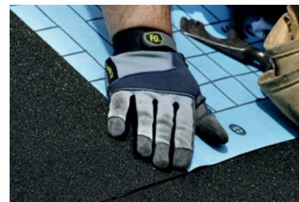
Apply Leak Barrier And Roof Deck Protection
